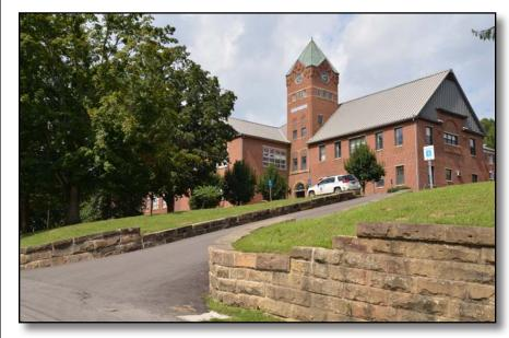
The cut-stone retaining wall that runs 450 feet in front of the Harry B. Heflin Administration Building has undergone reconstruction. The wall, which was originally built in 1936 by the Works Progress Administration from sandstone quarried from Nutter Run in Gilmer County, had been deteriorating and was posing some safety concerns.
