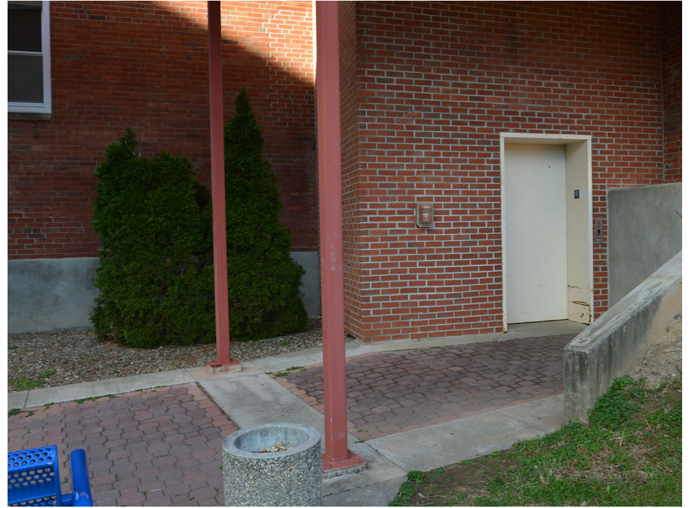
Access to the Administration Building/ Louis Bennett Hall elevator
