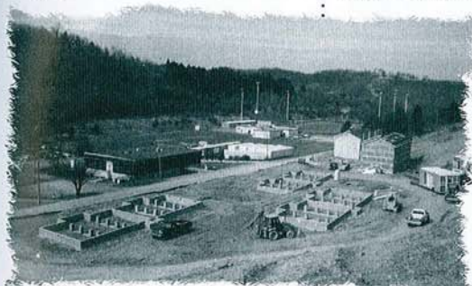
Pioneer Village foundations are ready to accept pre-built modules.
