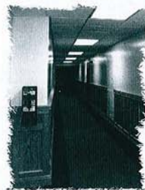
The Renovated hallway.
