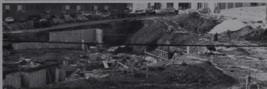
An overall view after some of the foundation and walls have been poured.
