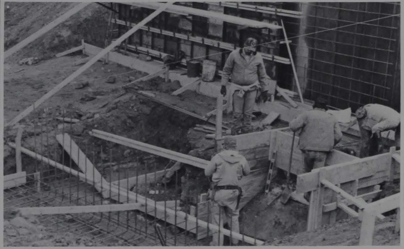
More preparation to pour the foundation for the New Fine Arts Building.
