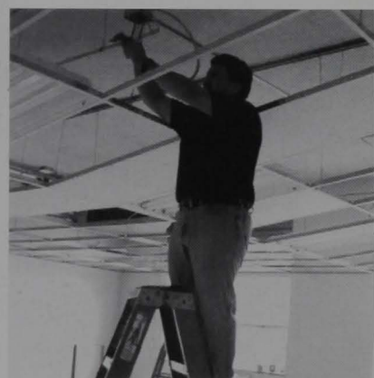
Below: Scott Lawson, Physical Plant Electrician, wires the lighting into the new drop ceilings.
