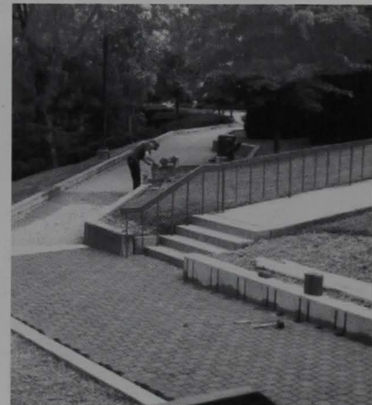
Below: Jim Tatman cuts brick to lay in the sidewalk.
