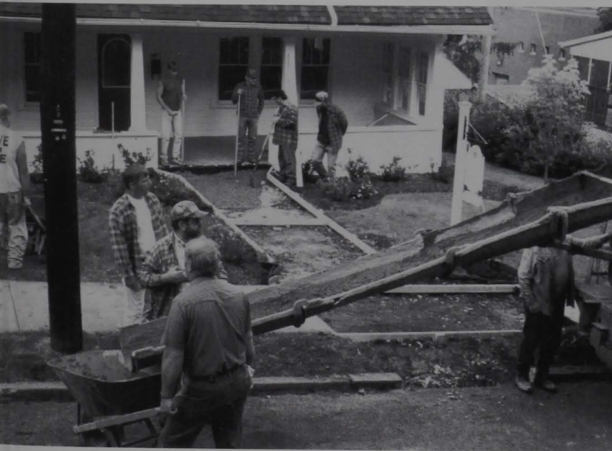
Left: Physical Plant staff meet the truck early to pour the new sidewalk for the Visitor's Center.
