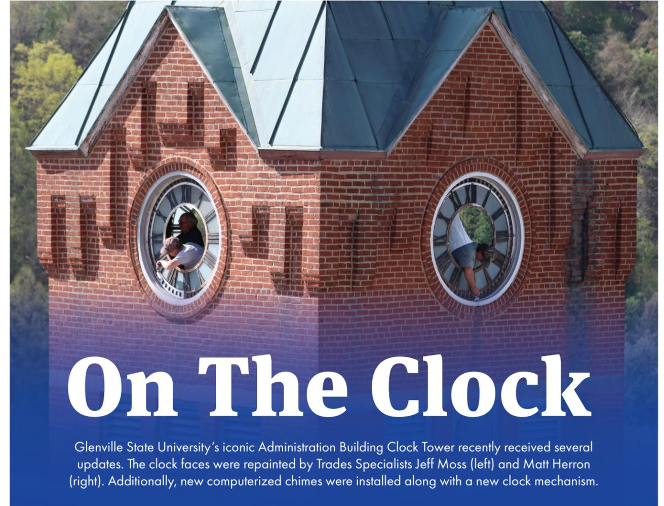
Glenville State University's iconic Administration Building Clock Tower recently received several updates. The clock faces were repainted by Trades Specialists Jeff Moss (left) and Matt Herron (right). Additionally, new computerized chimes were installed along with a new clock mechanism.
